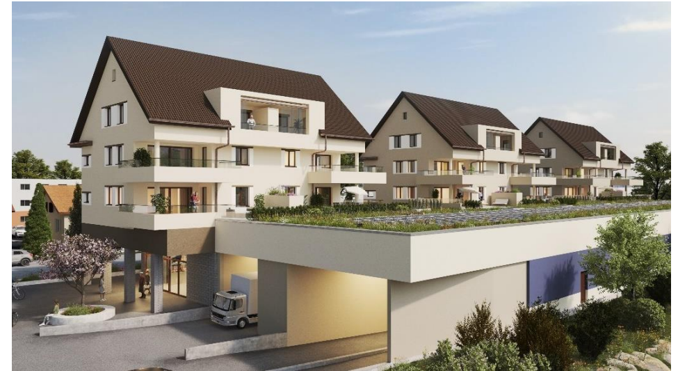
New build project Flawil south façade / Aldi customer entrance
