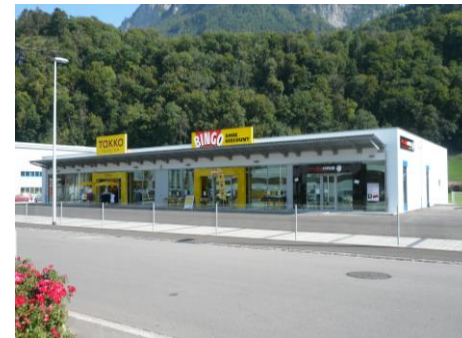
View of façade from main road (before)
