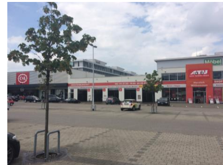
View of main entrance ATU
