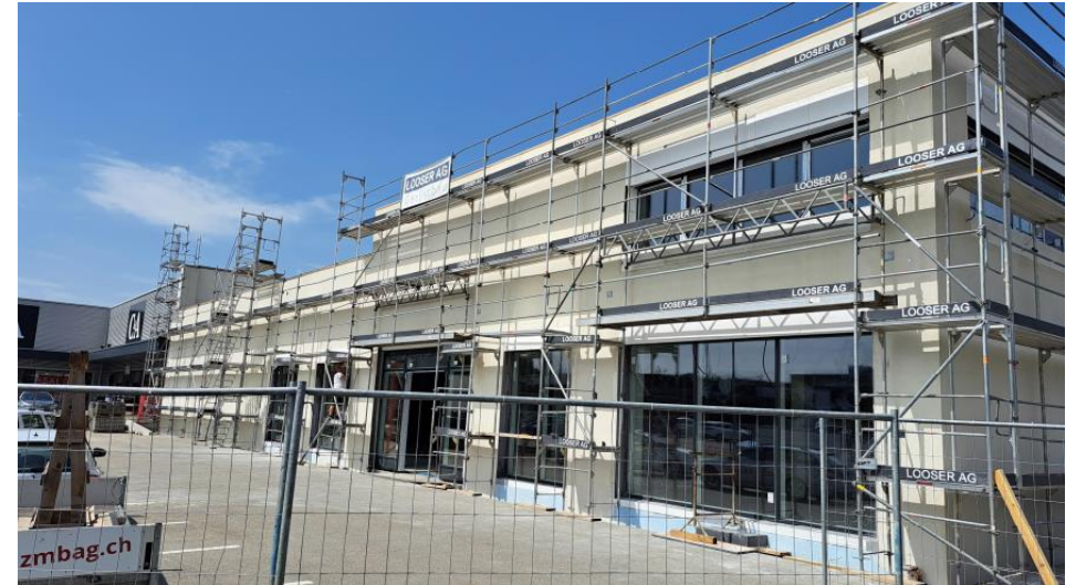
Main view with new entrance Müller Drogerie
