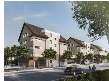
New build project Flawil north façade
