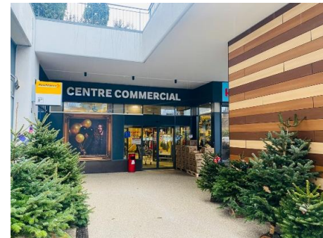
View of existing building
