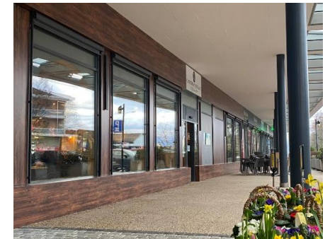
View of side of existing building
